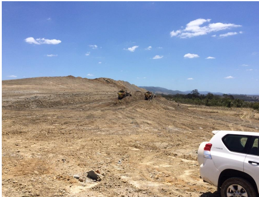
Photo: Bulk shaping on the Weismantel waste emplacement. December 2017.
