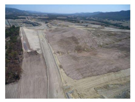
Photo: Bulk shaping and topsoiling at Weismantel waste emplacement and Duralie Haul Rd, taken Jan 2020.
