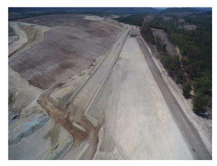
Photo: Bulk shaping and topsoiling at Weismantel waste emplacement and Duralie Haul Rd, taken Jan 2020.
