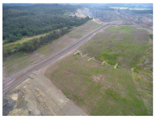
Photo: Bulk shaping and topsoiling at Weismantel waste emplacement and Duralie Haul Rd, taken Jun 2020.
