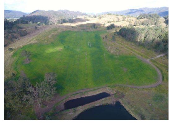
Photo: Shaping and topsoiling completed at Auxiliary Dam 1, Jul 2020.
