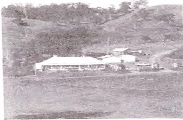
Eleven Mile Station, Black Soil - as it is today
